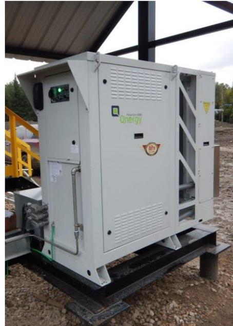
Further efficiencies can be realized by using waste heat (about 3 times the power rating) as a heat source for additional hot glycol.
