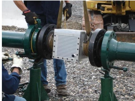
The generator outputs through an umbilical cable to its control box. This box can be mounted conveniently near the site batteries and or the supervisory control and data acquisition (SCADA) system for remote generator system-monitoring utilizing the existing SCADA system.
