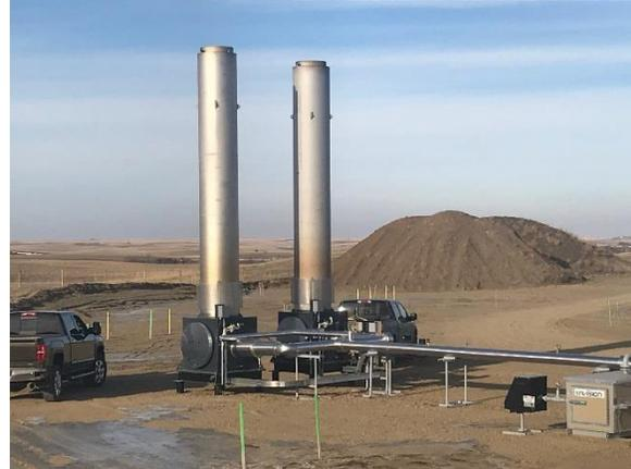
A small continuous pilot that uses less than 100 scf/d of fuel gas allows for stable combustion of intermittent flows as soon as the vapours enter the combustion chamber.
