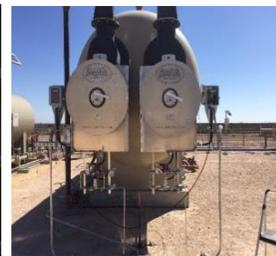
The Rush Burner's patented burner system achieves 99.99% total hydrocarbon destruction, and combustion efficiencies of 80% at pressures as low as two ounces. The Rush Burners can either use onsite power or the available solar package option. Incorporating safe and reliable ignition/flame sensing in the design creates a unique flame profile that increases heat transfer, inhibits flame lift off, and eliminates fire tube impingement. All Rush Burners come complete with:
